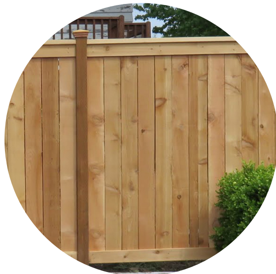
12 Perimeter board fence
